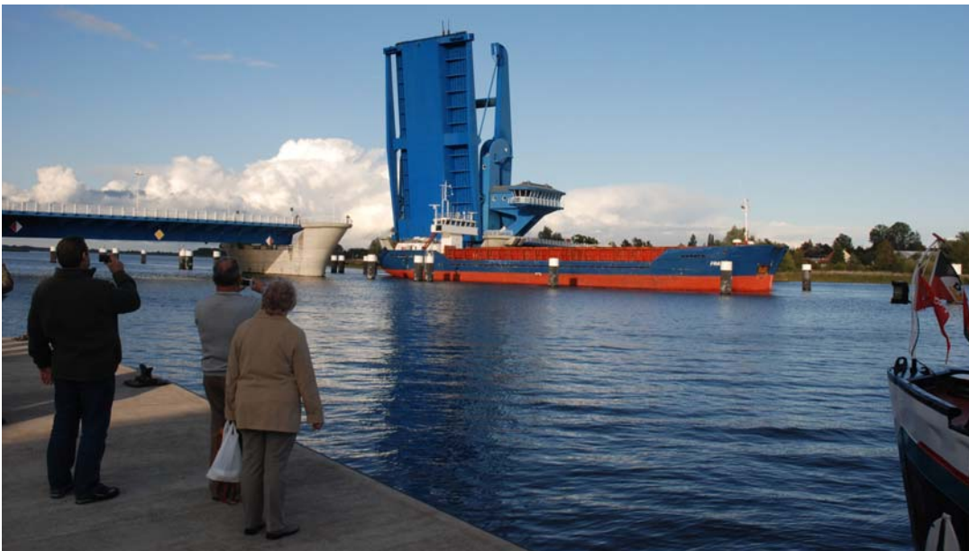
The Usedom Island lift bridge really does lift!
