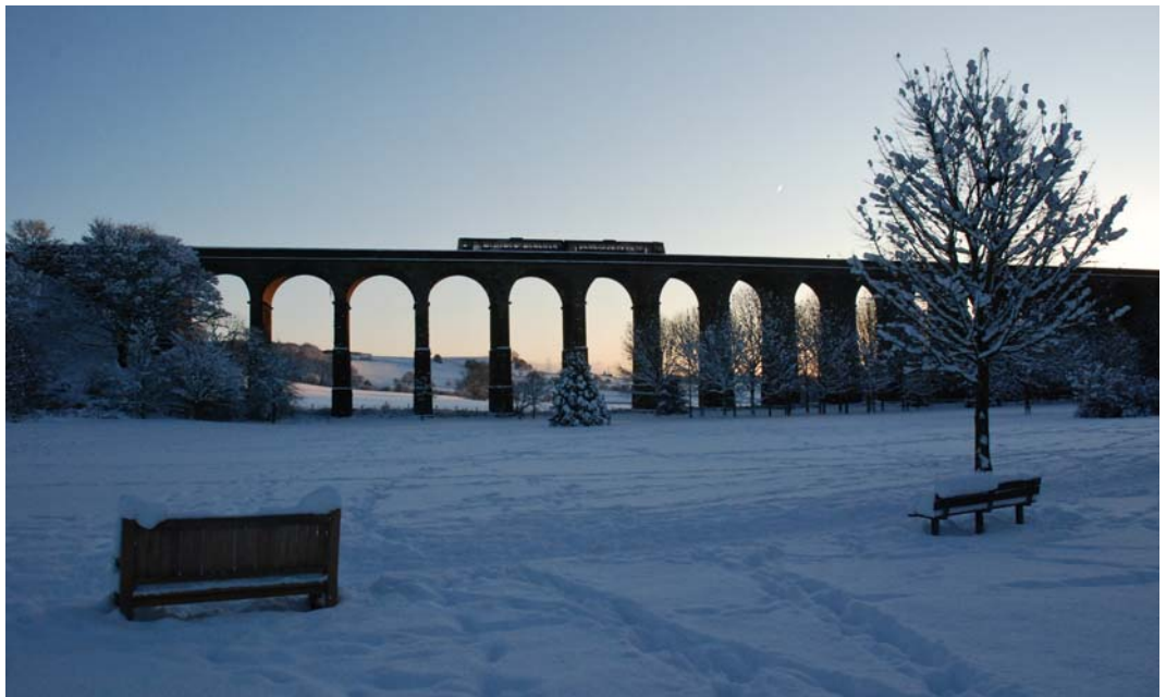
A train crosses Penistone Viaduct during the snow of November 2010
