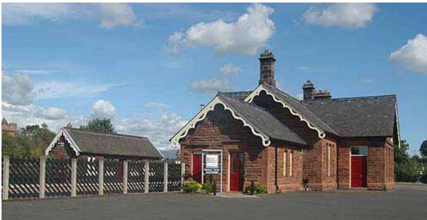
Lazonby Station used as offices
