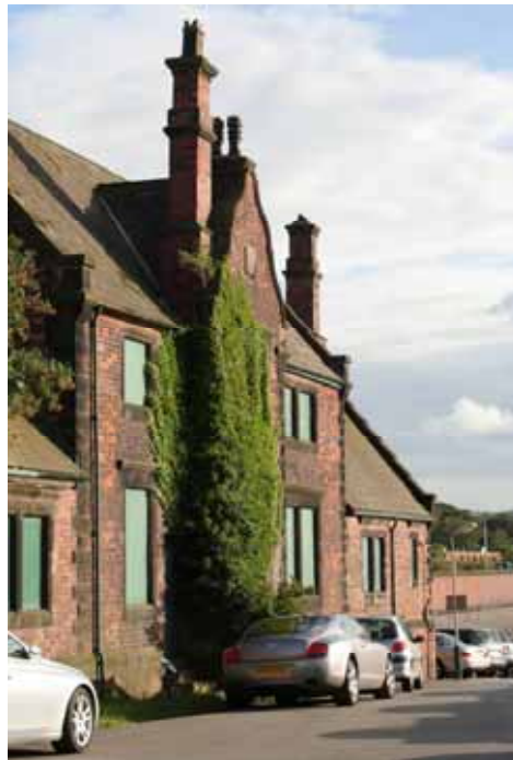
The boarded up station building at Frodsham (JMP Consulting)
